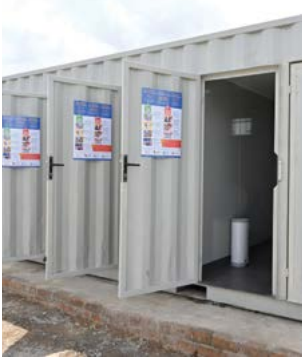
New-look loos: The Clear Enviro Loo full-flush toilets, being piloted in selected informal settlements, use wind and solar energy, taking the system completely off-grid. Recycled wastewater is used for flushing.
