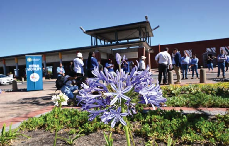
Ja, Kuyasa's busing again: Repairs and upgrades to the completely stripped and vandalised Kuyasa MyCiTi station in Khayelitsha have been completed. The station now again offers commuters and residents safe and easy access to reliable transport.
